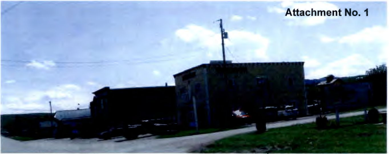
FACING SOUTH WEST
